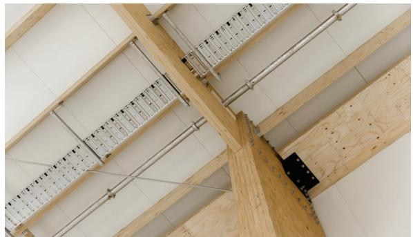
3 in 1. A roof, insulation & ceiling.
